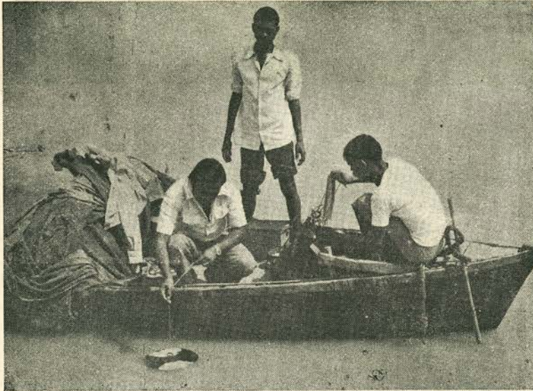
Fig. 6 Operating Secchi's disc for water transparency
